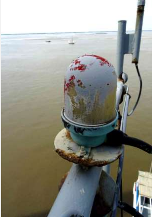
Navigation light cover was painted over
